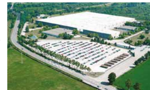
The Marelli Motori factory in Arzignano, northern Italy. Production moved back from Malaysia.
